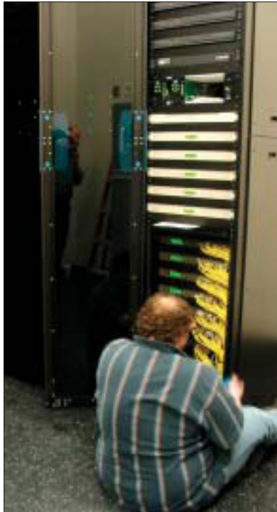
ACP Engineering Project Manager Mark Skrzypek works on data wiring at the base of a custom, 10-foot-high DVR rack. The project involved more than 250 DVRs.
