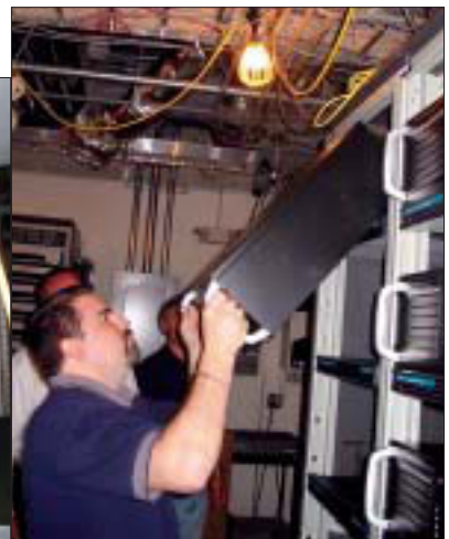
An installer prepares a rack to accept one of the Foxwoods project's 120 new American Dynamics DVRs, and later slides it into place. The units are kept in a room maintained at 68° F to avoid any thermal-related failures.
